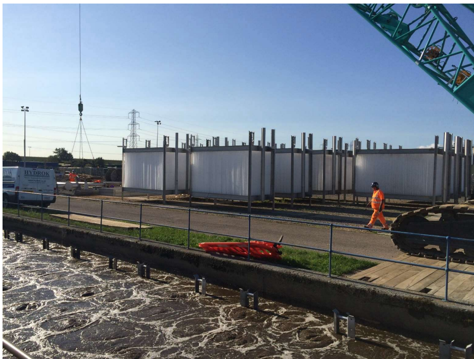
Figure 3 modular cages being assembled and installed
