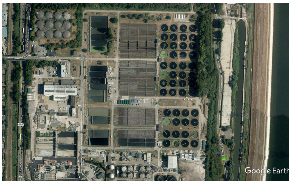
Figure 1- aerial view of Deephams STW before IFAS and Mecana
