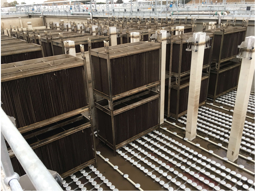
Figure 5 New A Stream 7m deep ASP, complete with transplanted cages from the old B Stream
